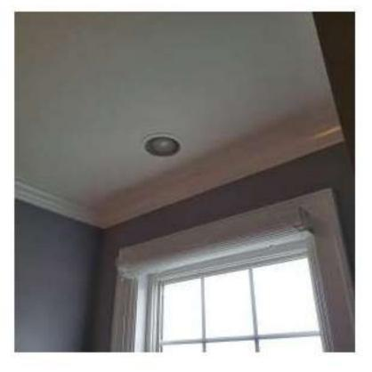
Ceiling fan in hallway bathroom on second floor would not turn on during testing
