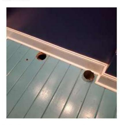
C. Recommend sealing hole in floor from wood knot near hallway bathroom on first floor
