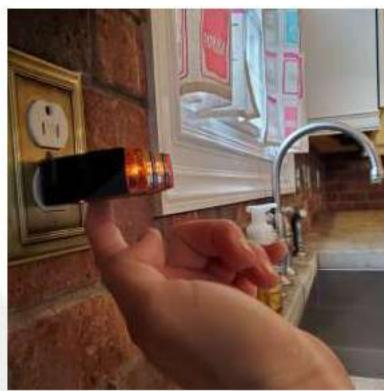
C. Outlet on right side of kitchen sink was reversed polarized (hot and neutral reversed)
