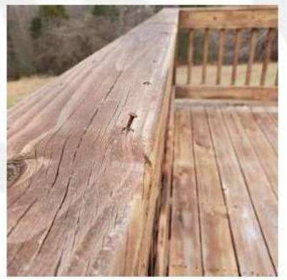
F. Nail securing railing to post on right side of back deck should be secured
