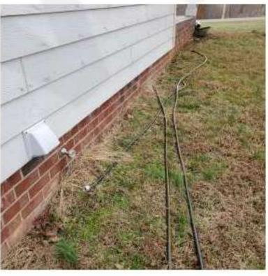
B. Exterior spigot near garage door on right side of house was Lewis and should be properly secured to siding. Spigot was not functioning at time of inspection
